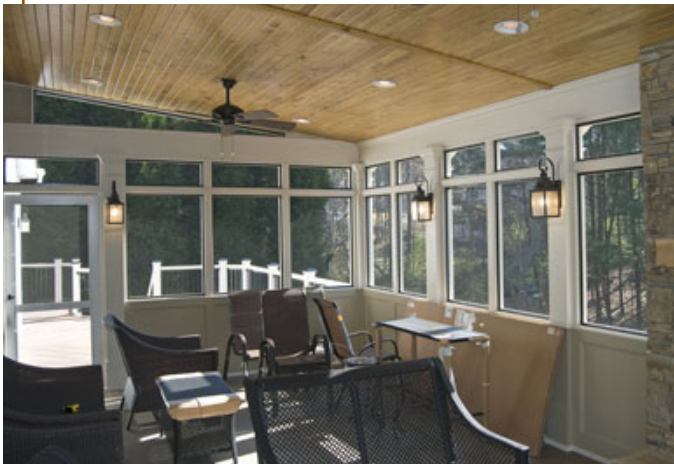
Figure 3. Complex projects like this screen room begin to look more like remodeling than deck building. A stable of good subs enables the author to take on a wide range of jobs.
